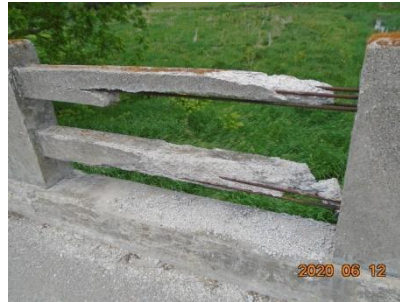
North Railing – Broken Rails
