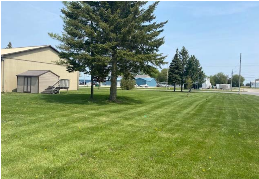
Figure 3. Site Photo showing general location of proposed addition.
