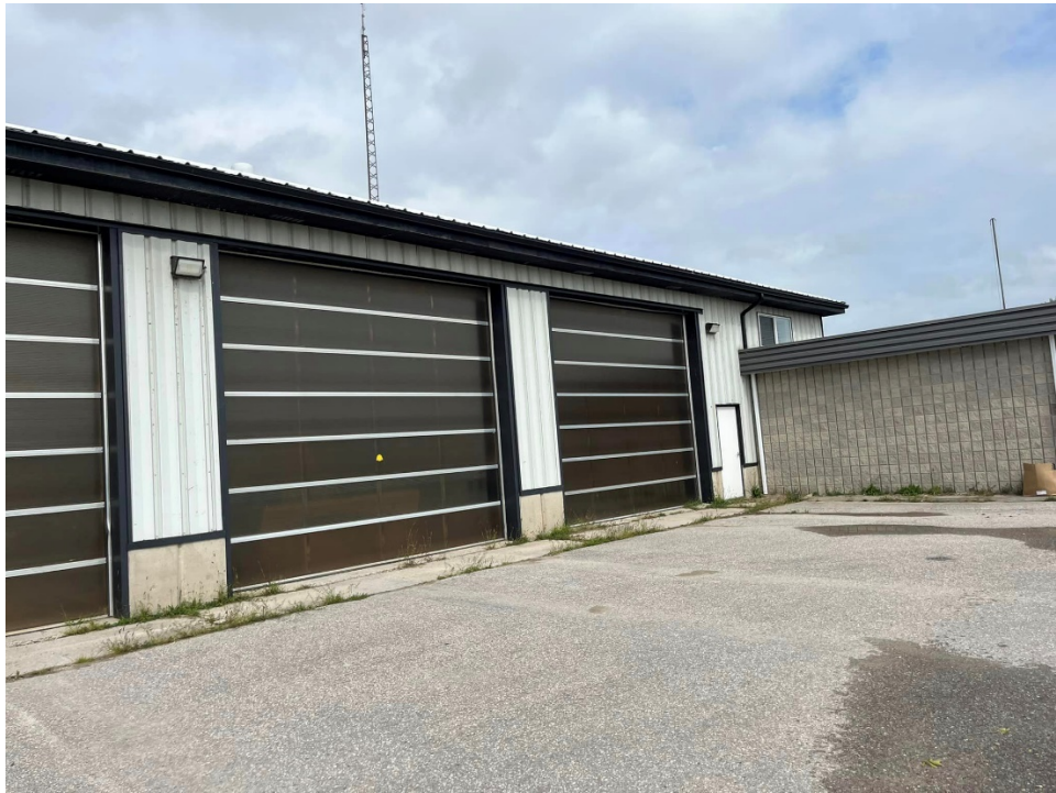
Grey Shop: New Trough and Repaired Soffit & Fascia
