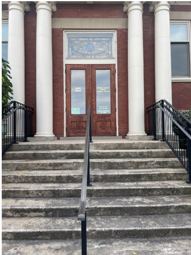
Seaforth Library: Refinished Front Doors
