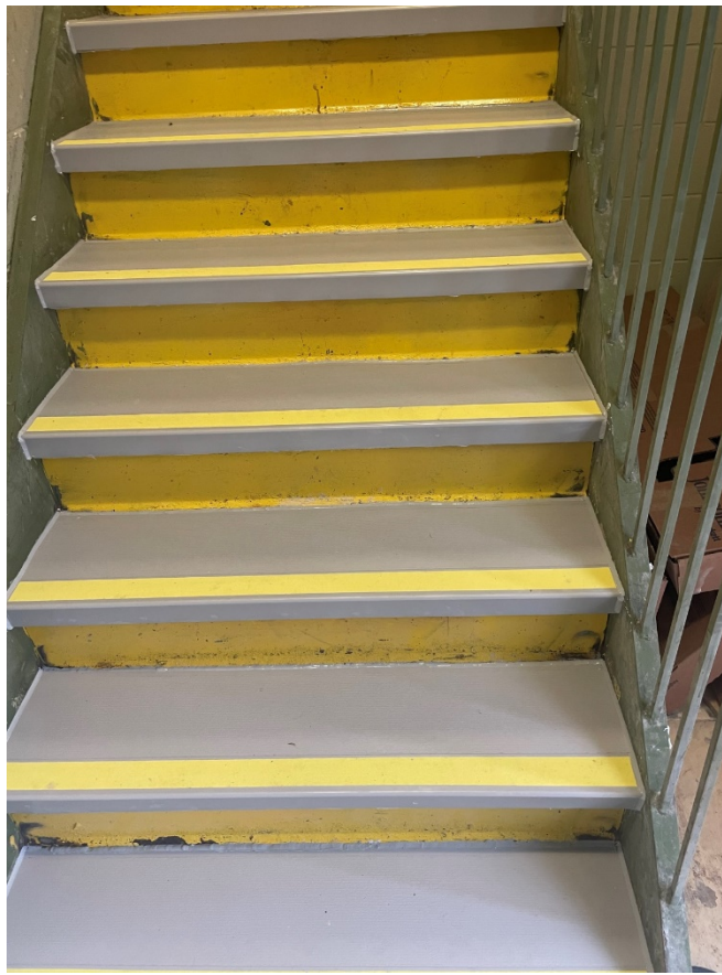
SDCC: New Vinyl Treads on the Back Stairs
