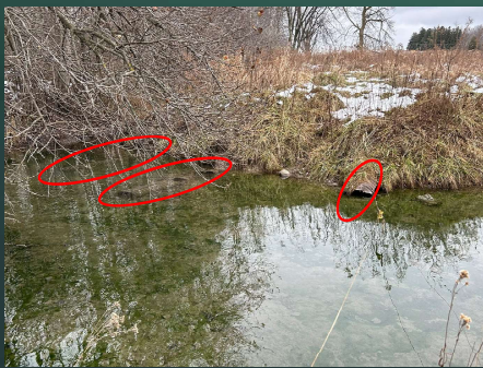
Existing Tile Outlets
