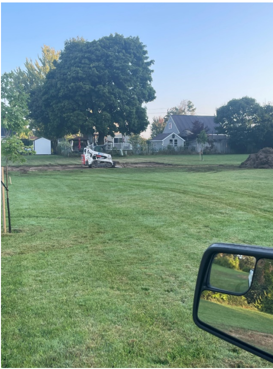
Starting the Excavation for the Concrete Pad
