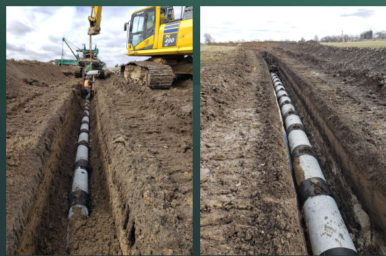
Tile Installation by means of Wheel Machine
