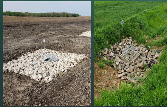
Catchbasin Installation
