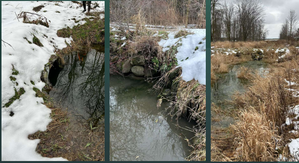
Existing Culvert Crossings
