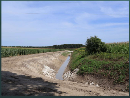
Typical Ditch Cleanout
